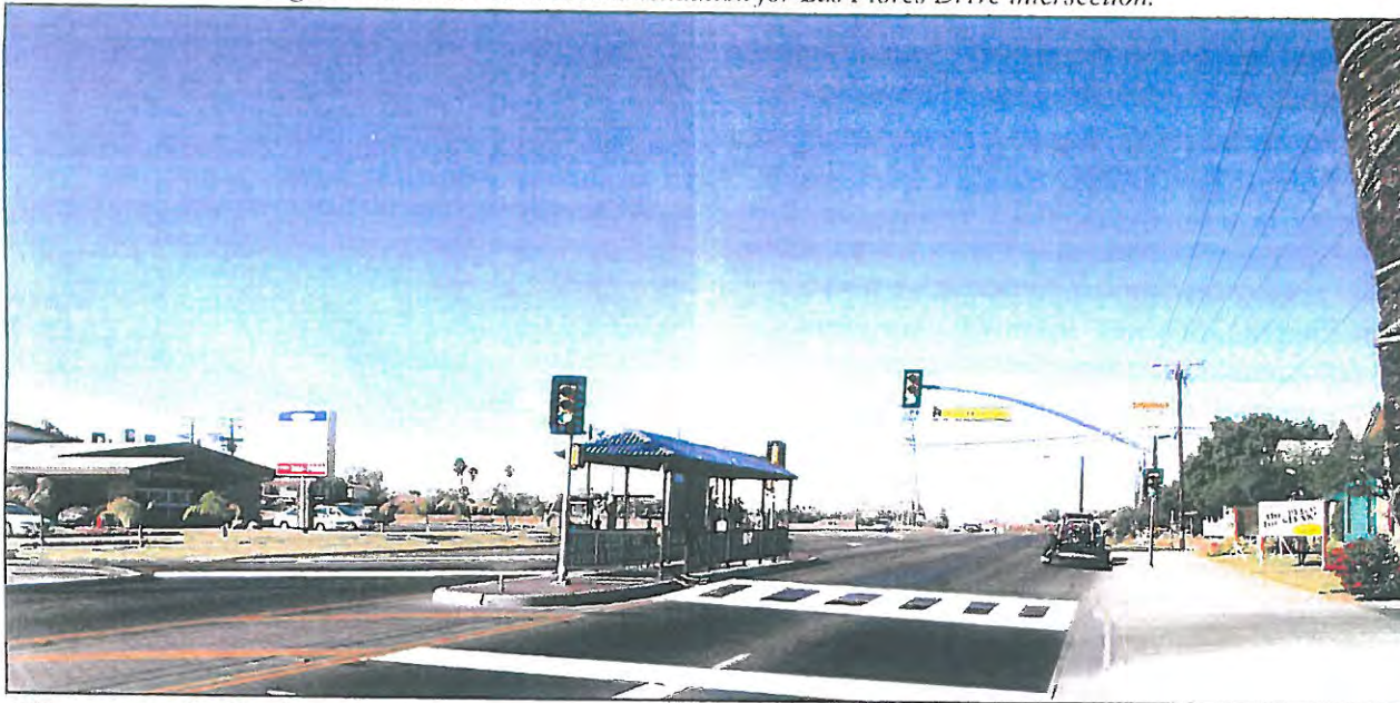
Offset crosswalks like this one on loan from Tucson, Arizona, force pedestrians to face oncoming traffic.
