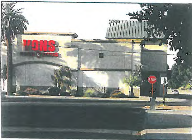
Marjorie Avenue does not line up with the Vons driveway...
