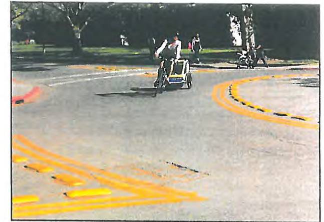
Low concrete pucks can enhance bike lane visibility.
