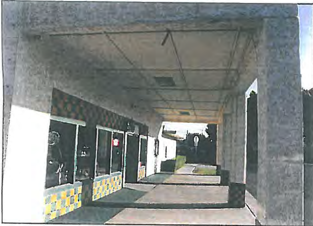
Plaza Park area commercial buildings.
