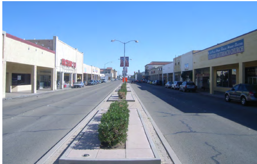
URM Buildings (Looking East Along Main Street)
