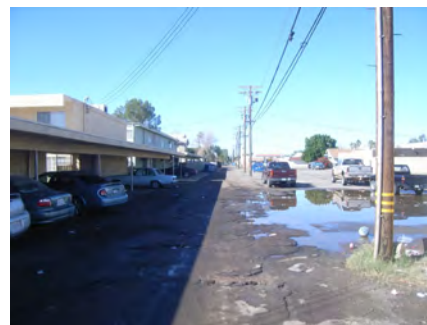
Parking at Rear Suffering from Disinvestment
