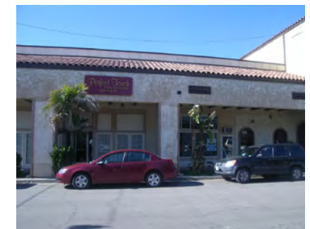
Parallel Parking on Side Street off Main
