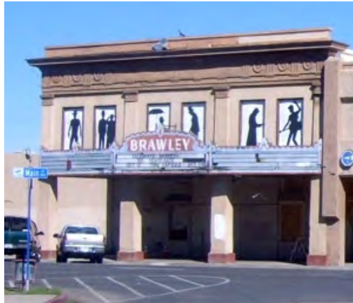
Historic Brawley Theater (Facade Only)
